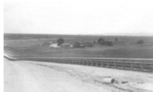
Figure 2: The Savmore overland belt conveyor.
